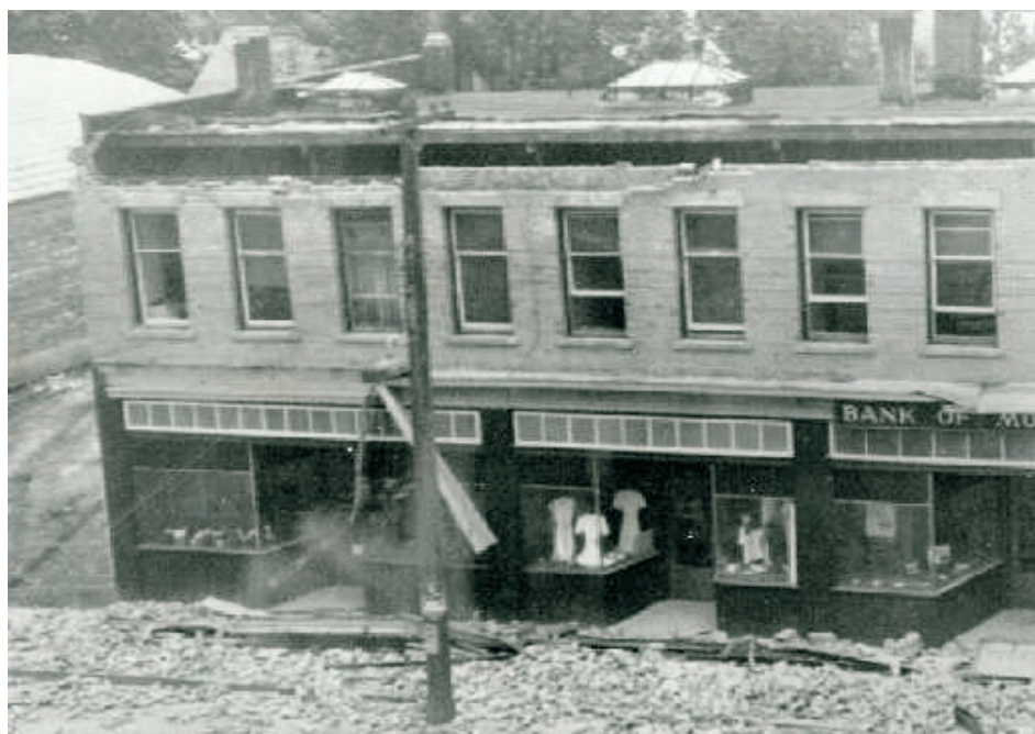
Figure 8. Damage to the Bank of Montreal building in Port Alberni, BC, resulting from the M 7.3 earthquake of 1946.
